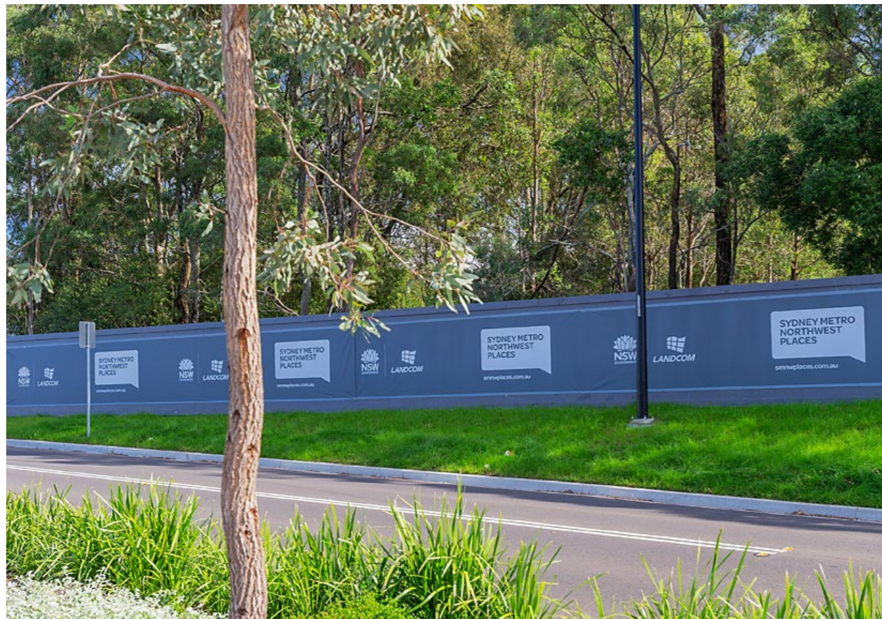
Example branded banners installed on timber hoarding.
